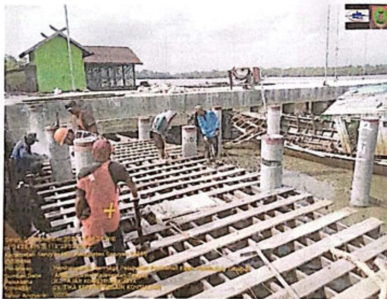
PEKERJAAN PEMOTONGAN TIANG SPON PILE
