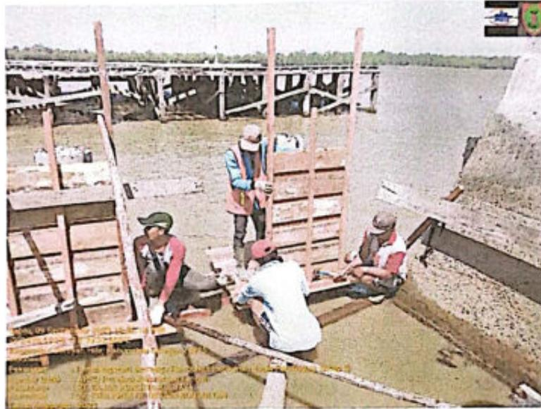
PEKERJAAN BEKISTING BALOK FENDER
